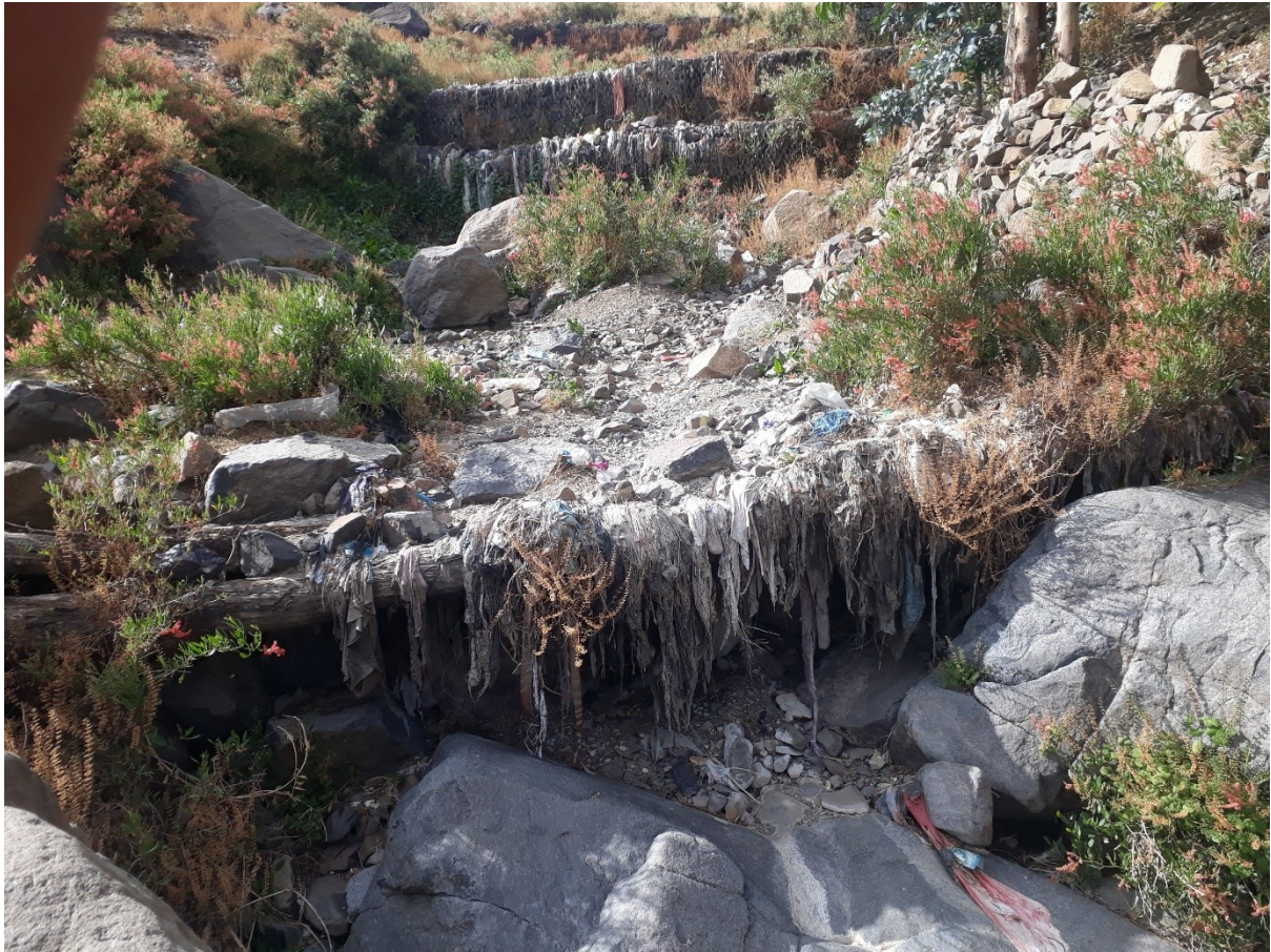
Figure 27. In the Harena torrent, that drains Hagere Selam to the east, the log dams (constructed in 2011) [25] have some of their woods rotten away, but the clusters of large rocks behind them are standing strong, which leads to storm runoff that is better spread over time. The technique in itself has proven its cost effectiveness, but this is also related to the fact that the gully upstream from those check dams has been fully treated with gabion check dams. And more upstream, a large gravel dam buffers floods. There has been a maintenance campaign in places where it started to collapse – that was before the war. Inside and along the gully the vegetation is regrowing. The amount of garbage in the deposits is unprecedented and related to absence of waste collection in Hagere Selam during war and blockade.
