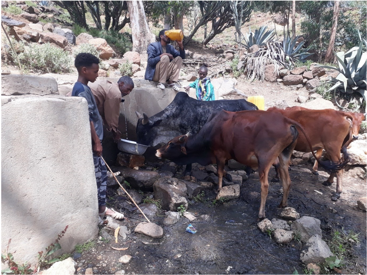
Figure 28. A dysfunctional spring development in May Toqem in November 2023. There had been several spring developments there, and the Selam Watsani project [59] built the latest chamber and taps in 2012. The taps are not working anymore, the cattle trough below it is not operational either; the water is taken directly from the overflow of the storage tank and people use it there both for livestock and domestic consumption. Already before the war it was common to see such dysfunctional or abandoned spring development projects. Additional impacts by the war and the lawless period are diverse and shown below.
