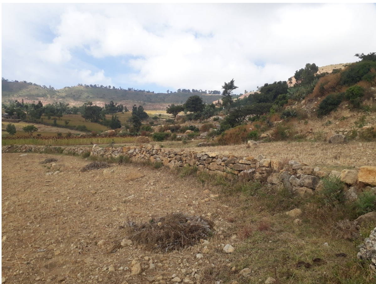
Figure 16. In the Argaqa area, all stone bunds, constructed in the years after 2000 [22, 23], were intact in October 2023. Overall, among the representative sample of 31 observed stone bunds (Table 2), 25 are in acceptable to perfect condition, four have collapsed in their upper part without generating concentrated runoff and two need rebuilding. Bunds built from limestone and sandstone are particularly in good condition (Figures 13 and 16), while those built from basalt require much more maintenance (four out of nine observed), which is clearly related to the irregular, often spherical shape of the rocks (Figure 14).
