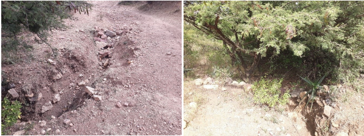
Figure 5. Along the rural road to Addi Qoylo gullies have occurred due to a lack of road maintenance since 2020 (left, looking upslope). The runoff path then leaves the road and enters into an enclosure managed by the “Trees For Farmers” [64] project (right, looking downslope). Though no salaries or payments were received during the war, the guards have continued protecting it and the enclosure stands nicely. The enclosure totally buffered the runoff coming from the road and the gully is discontinued and sediment is deposited. Photographs taken in November 2023.
