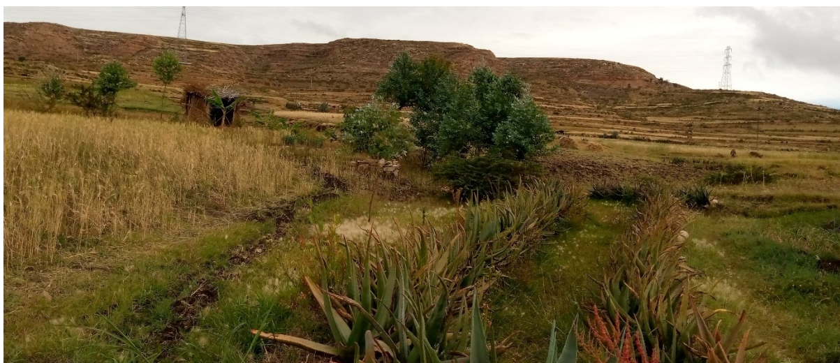
Figure 32. The previous May Bi'ati gully where subsurface dams were installed in 2011 [56] has become a linear oasis, as observed in November 2023. The works led to a near-total fill of the gully (in the middle of the photo) and a raised water table; in the war period, ten farmers have done the effort to irrigate the rehabilitated gully bottom and adjacent lands.
