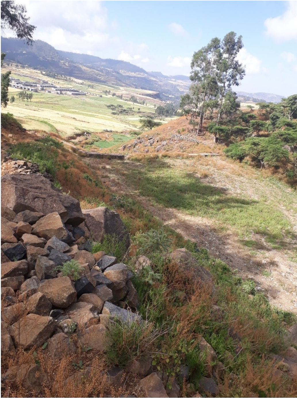
Figure 25. In a gorge at the southern side of Hagere Selam a large flood buffer dam had been constructed that got rapidly filled with coarse sediment [42], which reduced peak flows and enhanced infiltration. In the downstream area, around 1999, very active gullying occurred (Figure 26). After construction of the dam, soil conservation works and abandonment of free grazing, the gully downstream has become a linear oasis; in October 2023, there were quite some locations in the previous gully channel with ponding water. There is good grass growth, and also good discharge in the river downstream.
