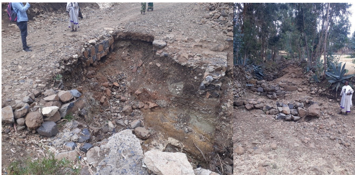
Figure 24. Downslope from Maltmasha, the road from Dingilet to Hagere Selam is affected by gully incision (left), which originated in 2021. The footpath that runs in the thalweg on the upper side serves as a waterway during storms [50]; it is equipped with steps and check dams at regular intervals, which were not destroyed, while the floods have simply cascaded over it (right). The increased storm runoff comes in response to the establishment of the new settlement at Maltmasha. The conflict of interest is that from a management point of view the footpaths should not concentrate the runoff, yet in the village and immediately downslope, dwellers and farmers just want the footpath to concentrate the runoff and evacuate storm water as fast as possible with gullying as a consequence in downstream areas. Such situations are already difficult to manage in peace times, but during the war the community was less organized and the remaining regional and village authorities did not at all focus on spatial planning. Photos in October 2023.
